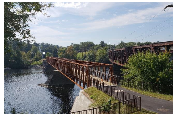
The new walking bridge holds critical water and sewer mains...and provides a convenient way to get some exercise and pay your water bills at the same time!
